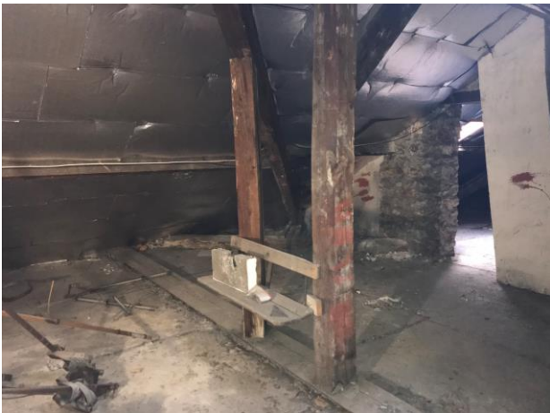
Figure 7 : Vue ensemble combles - R+3
